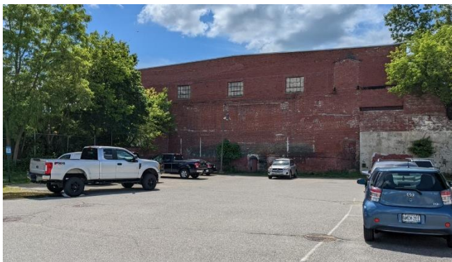
Figure 9 Paved Storage Lot
